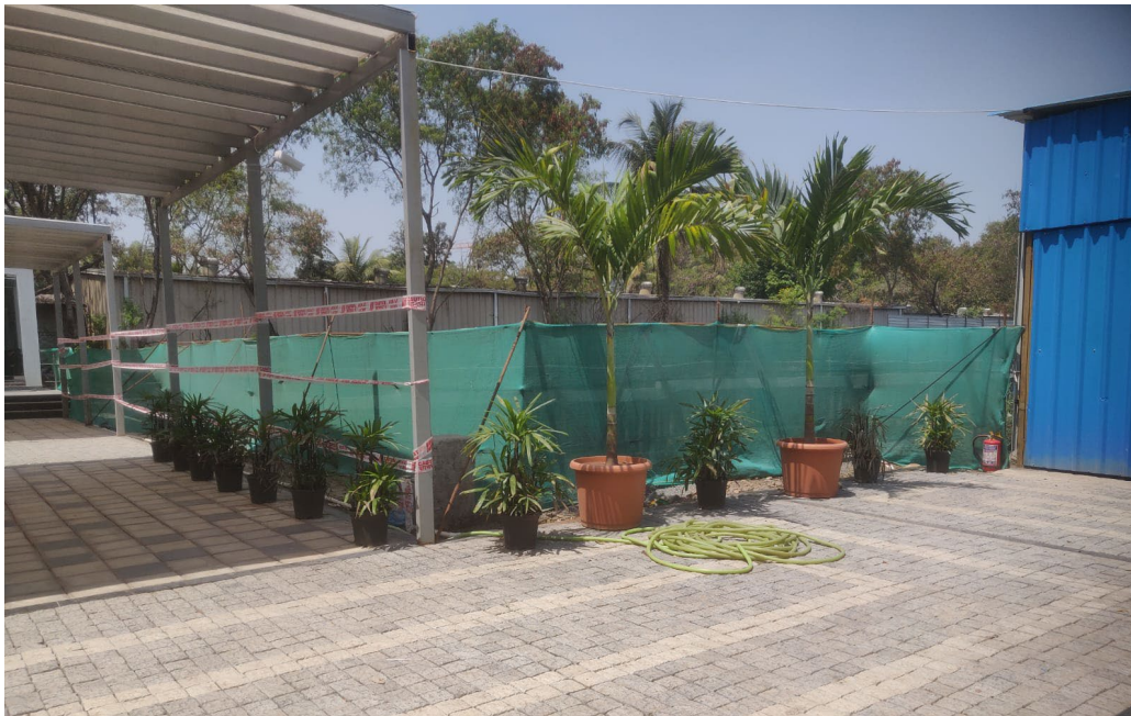
TREE PLANTATION AROUND SITE OFFICE 2
