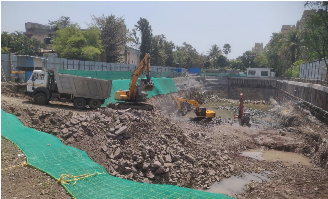
CURRENT SITE STATUS
