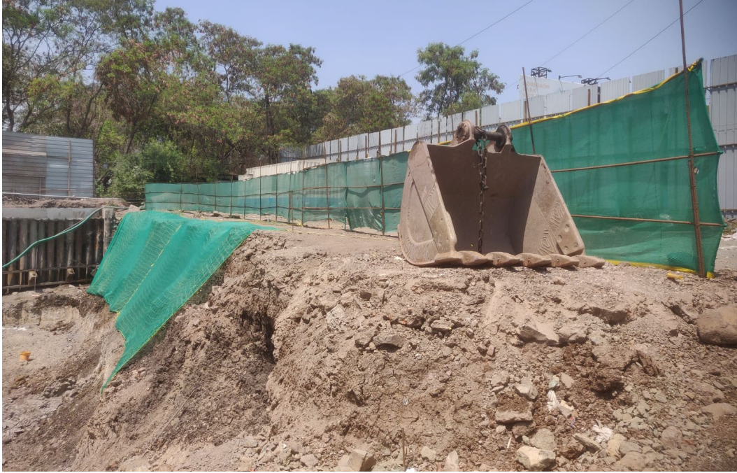
EXCAVATION SIDE PROTECTION
