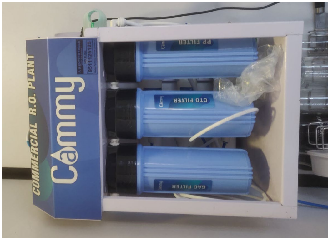
RO PLANT FOR DRINKING WATER FACILITY
